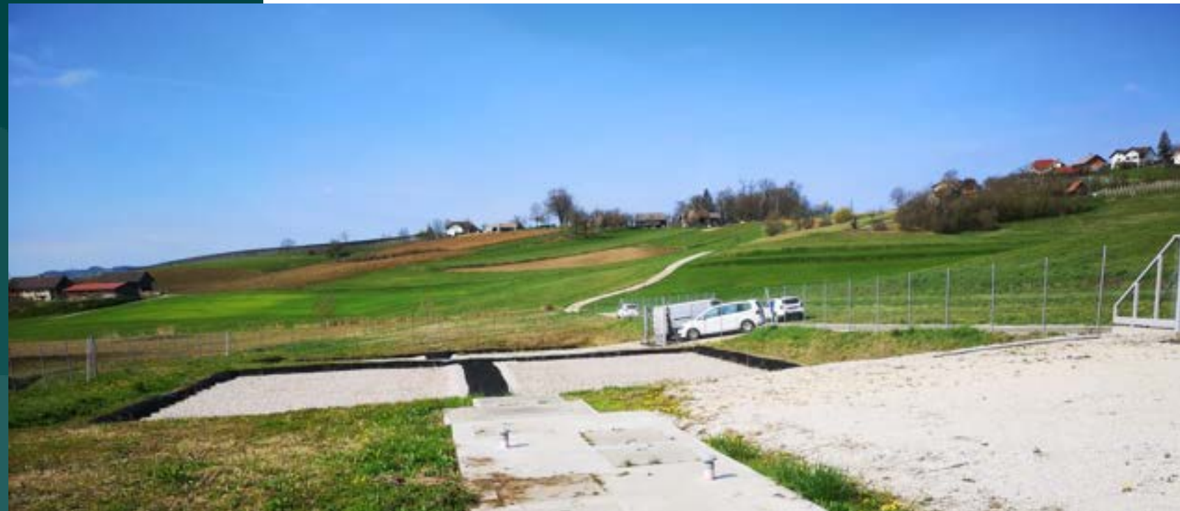
Constructed wetland and sludge drying reed bed Raka, Slovenia (400 PE)
