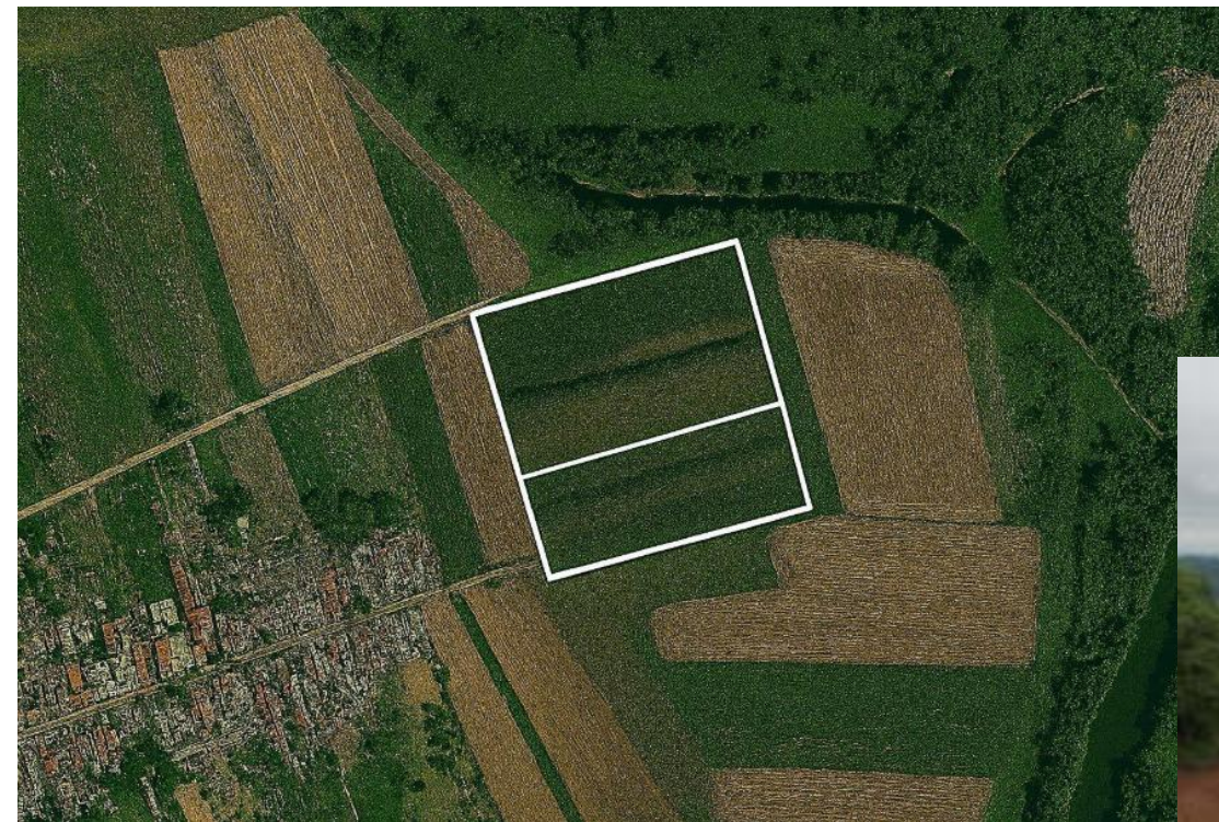
Constructed wetland Gložan, Vojvodina, Serbia (2.200 PE)
