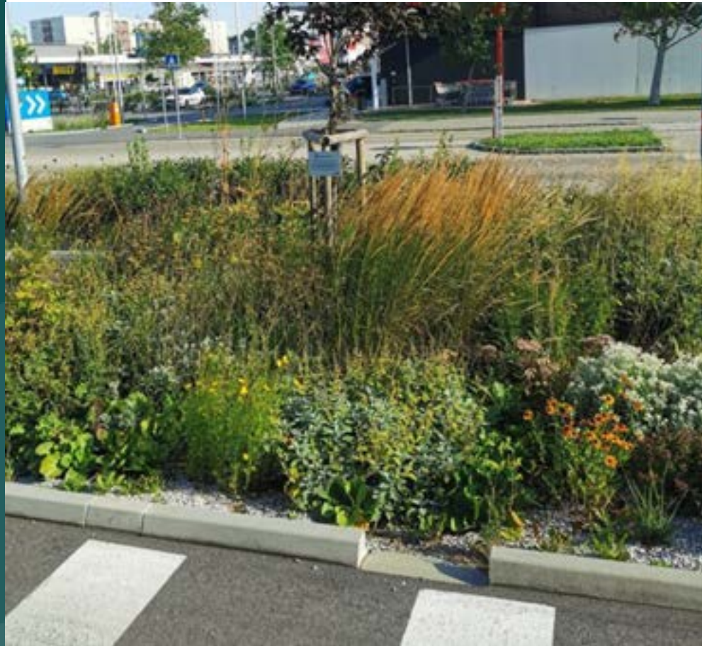
Raingarden for surface runoff retention and treatment, Austria
