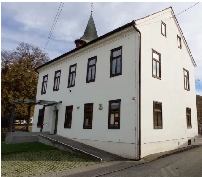
Picture 3: Smart Charging system will be set up at the extension roof of the Smart house - in the Biofuture center
