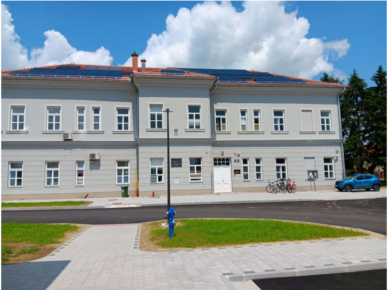
Figure 2. Administrative building in Knowledge Centre of Medjmurje County in Čakovec– PP4 Pilot site
