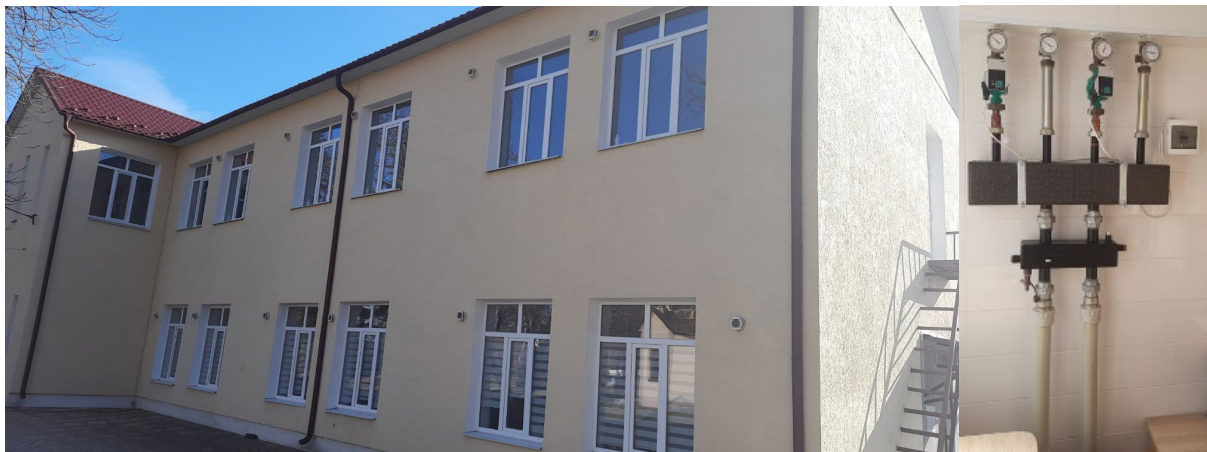
Figure 3: Place of installation of the heat pump
