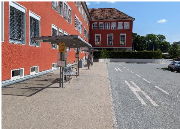
Insufficient weather protection at waiting areas (Bus station in Stegersbach/Austria). Credit photo: © Andreas Friedwagner
