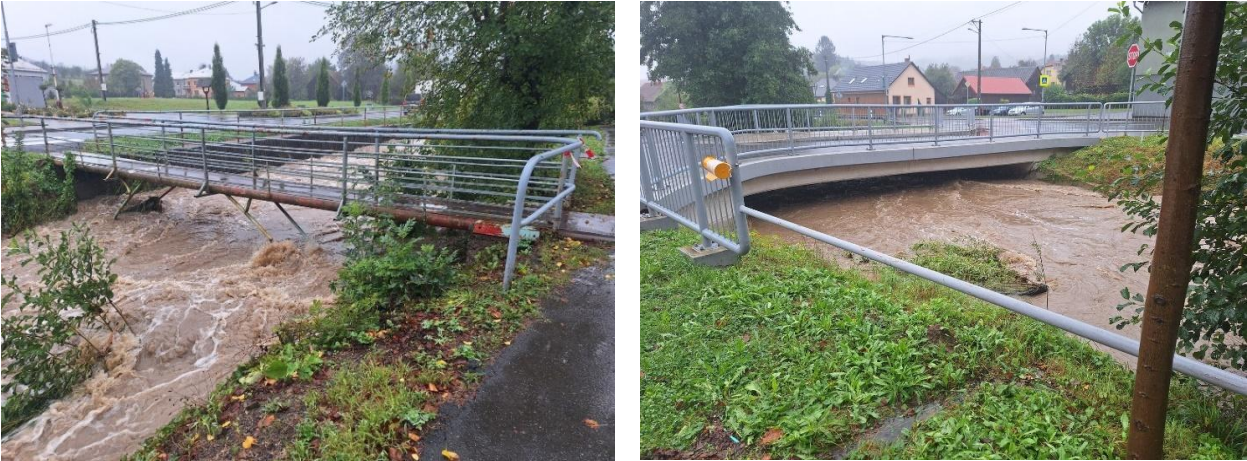
Figure 15: The bed of the Ratibořka stream, designed for a flow of Q_{1000} , was almost full on September 15-17, 2024 (Source: Archive of Ratiboř, 2024)
