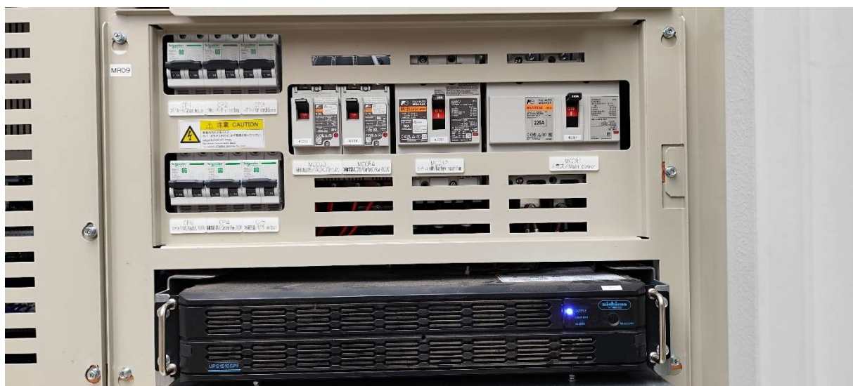
Electrical panel and control hardware for the NAS battery system
