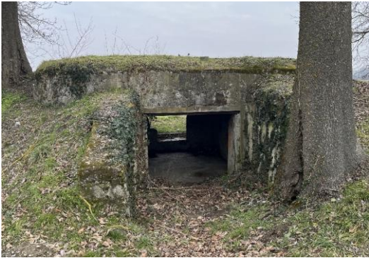
Border Fence period - bunkers
