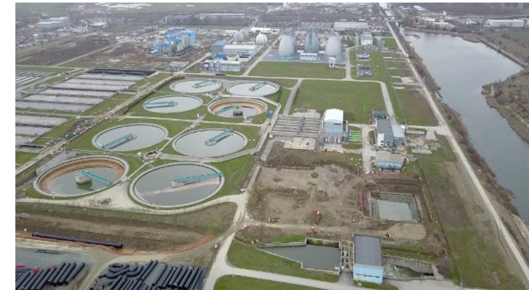
WWTP Glina, Bucharest, RO
